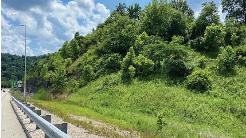
Jackson Gateway: Existing Road Cut (Before)
