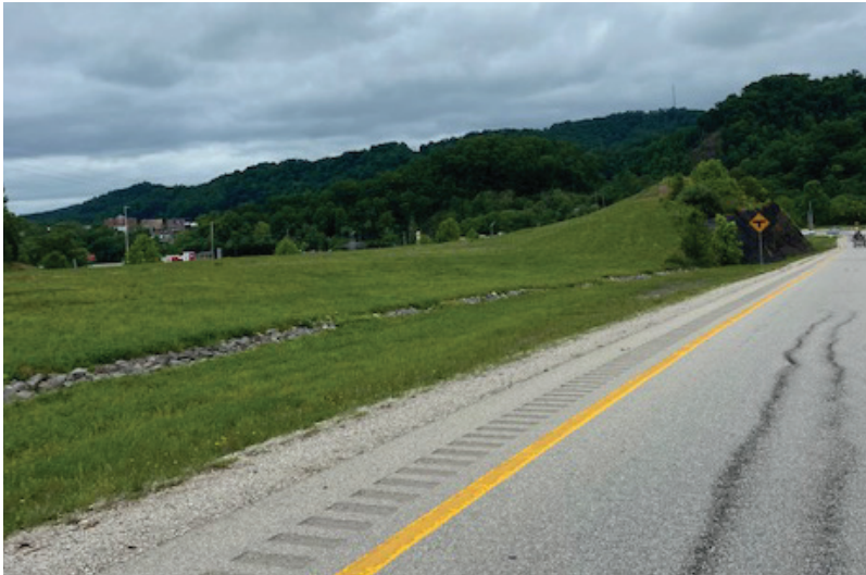
Jackson Gateway: Existing Road Cut (Before)
